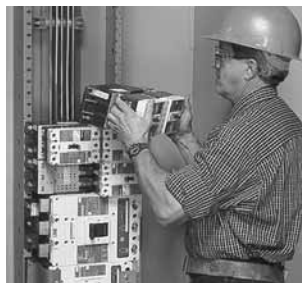
Panelboard Installation
