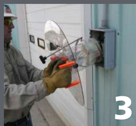
3 Removing/pulling meter
