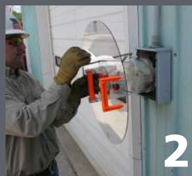
2 Closing non-conductive jaws with actuating rod
