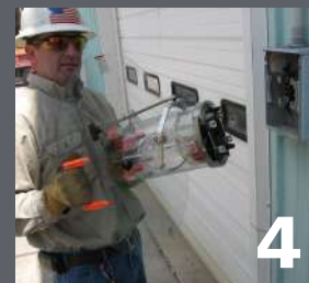
4 Meter removed from socket base
