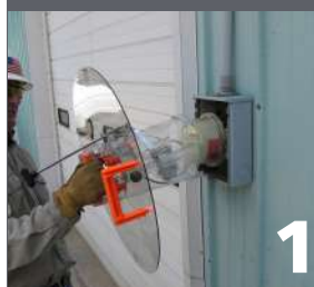
1 Positioning on residential meter
