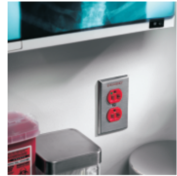
Emergency power areas must be identified as such with distinct marking or color on wallplate or device
